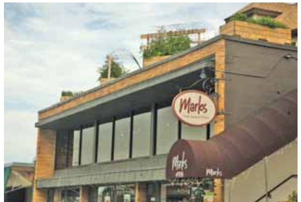
View of roof top garden from street level.
