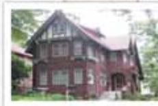
Doyle Home 903 Mercer Boulevard
